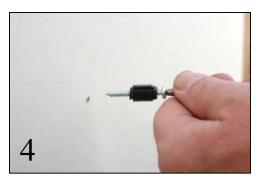
Screw ratchets to wall at marked locations. (#8 screws recommended)
