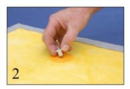
Insert marking plugs into the Snap-On anchors.
